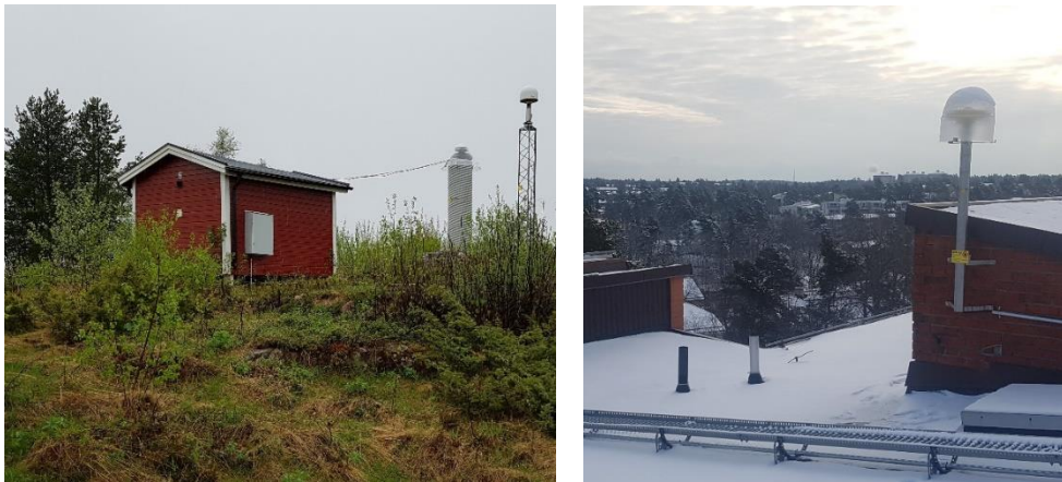
Figure 1: Sveg is one of the SWEPOS class A stations. It has an old monument (established in 1993) as well as an additional monument (2011). Right: Gustavsberg is a SWEPOS class B station with a roof mounted GNSS antenna established mainly for network RTK purposes.
