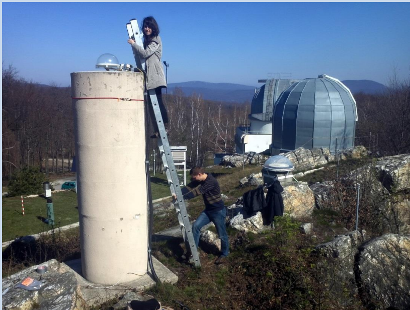
MOP2 (EPN STATION)
