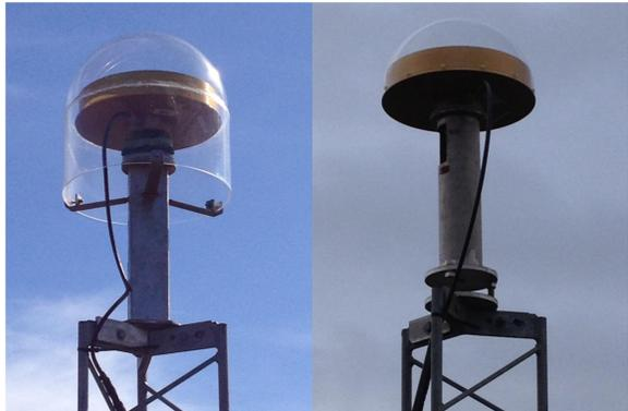
Figure 1: OSOD-radome to the left and OSOS-radome to the right. Photo: Johan Löfgren, Onsala Space Observatory, April 2015.
