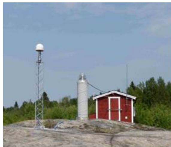
Figure 3.1: Hässleholm is one of the SWEPOS stations belonging to class A. It has both a new monument (established in 2011) and an old monument (from 1993).
