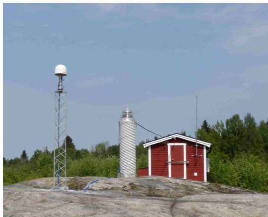
Figure 2: The SWEPOS station Hässleholm with the new and the old monument.
