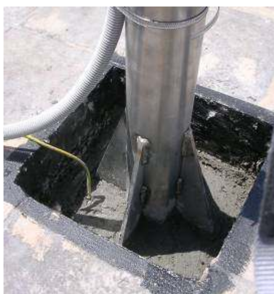
Figure 4: Typical procedure for the installation of a HEPOS station on the roof of a building.
