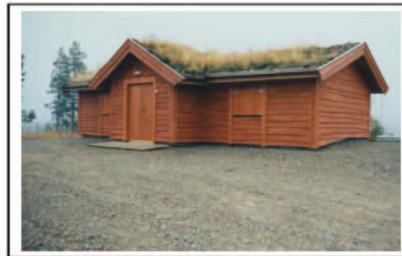
Outside view of the station during measurement
